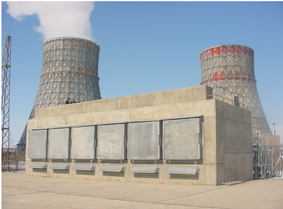
Picture 2. Dry Spent Fuel Storage Facility
